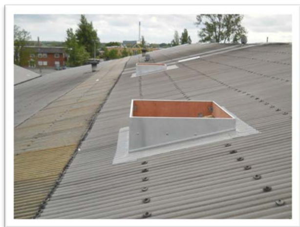
Example of base on sloping roof
